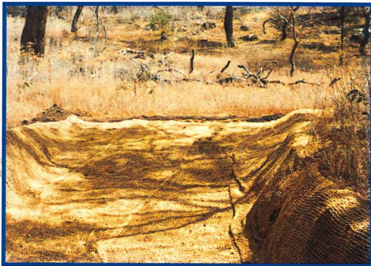
Erosion control and regeneration go hand in hand. Regeneration always has a role to play in erosion management. The before and after shots here show treatment in a creek bed site where gully erosion was active and tunnel erosion a threat. The first shot shows forming and lining the creek bed. The second shot shows the same site which was fenced, four years later, in a stable condition. Native grasses were broadcast here and shrubs were planted from tube stock.
